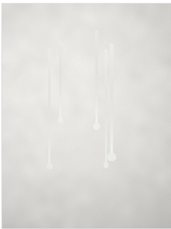
Paint finish over the affected section
